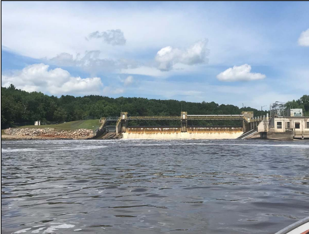
Photograph 2: Facing upstream toward BPU facility, including tainter gate (on left) and bascule gates (on right). Water is currently flowing over both bascule gates (July 16, 2019).
