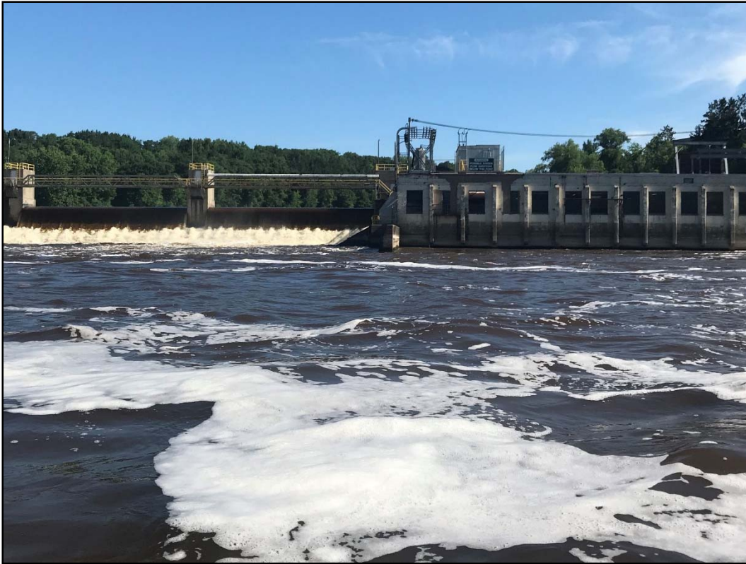
Photograph 1: Facing upstream toward BPU facility, with bascule gates visible on the left and the powerhouse visible on the right. Foam on water surface is caused by naturally-occurring tannins in the water (July 11, 2019).
