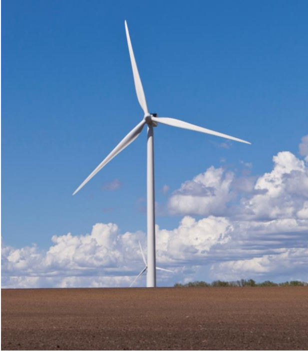
Minnesota Municipal Power Agency Oak Glen Wind Turbine Blooming Prairie, MN
