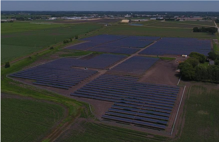
Southern Minnesota Municipal Power Agency's & Center Municipal Power Agency/Services' 5 MW Lemond Solar Center Owatonna, MN
